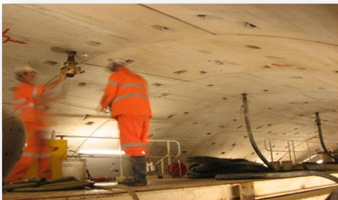
Figure 4 Secondary grouting of every second segment (courtesy Mr. Michael Huber) and potential insignificant primary grouting (Image modified from [11])
