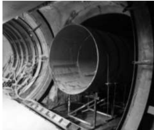
Figure 6: GRP installed in adit.
