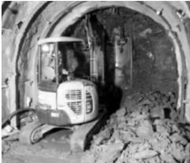
Figure 5: Adit excavation and ground support.
