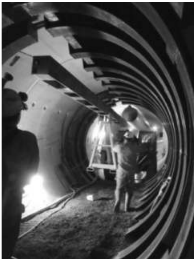
Figure 4: Installation of temporary support at adit.
