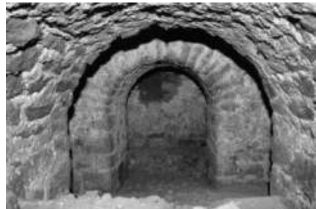
Deep, dark secret: The tunnel that was discovered recently in the 144-year-old building of the Sassoon General Hospital. Pic/Krunal Gosavi.
