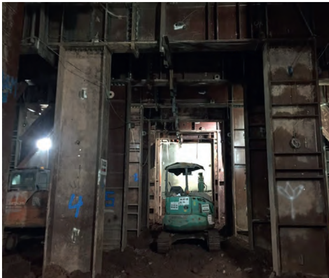
Fig 8. Site constraint for movement of excavators
