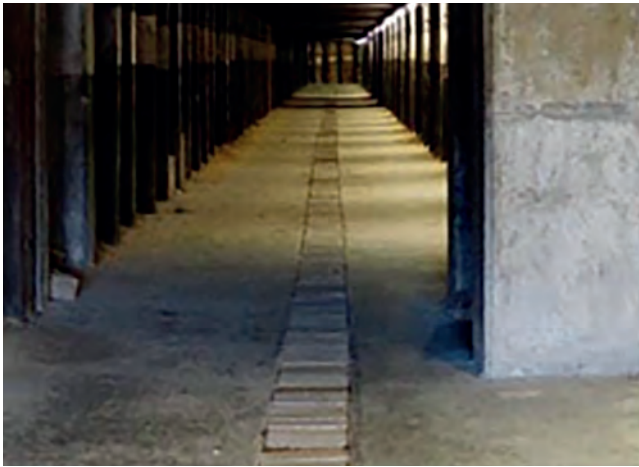
Completed timber supports 1942. As installed in Dogleg Tunnel on Cockatoo Island by MWS&DB in September/October 1942
