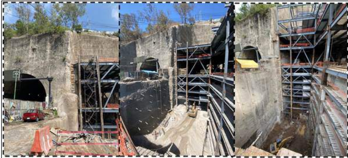
Figure 18. Pictures of the different excavation advances with proposed confinement system
