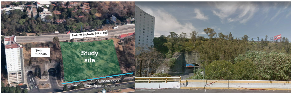
Figure 2. Graphic description of the site and photograph of conditions before construction
