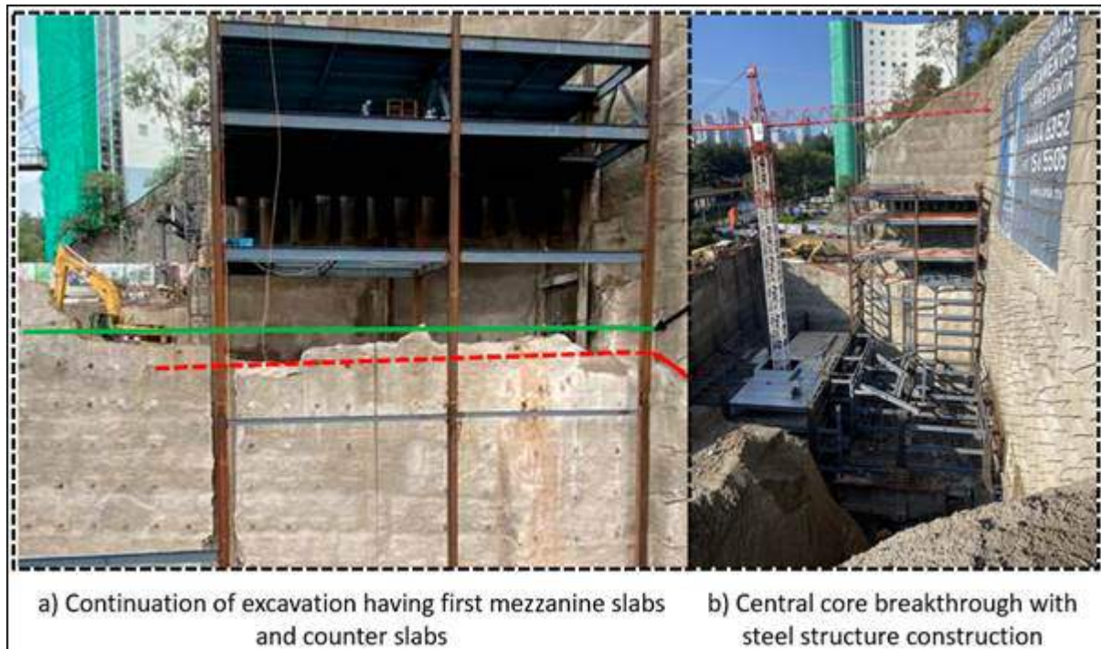
Figure 17. Continuation of excavation and construction of shoring system
