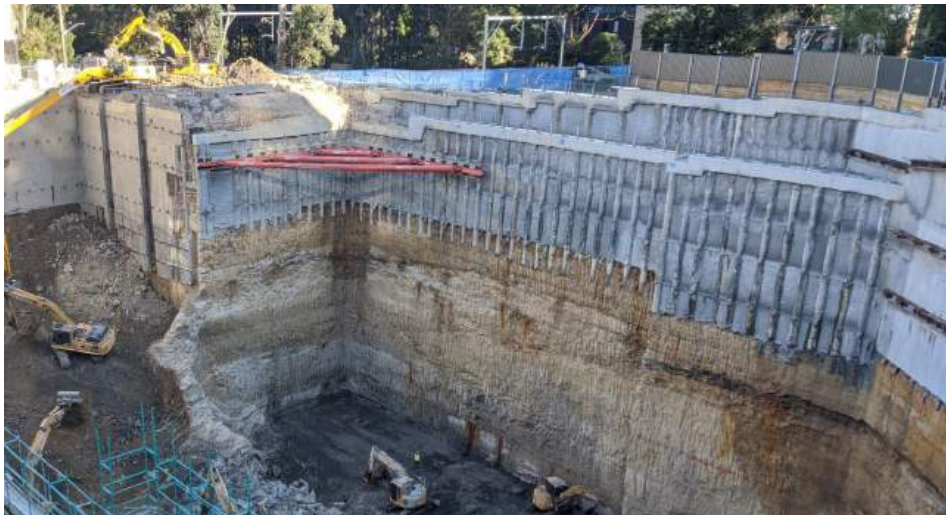
Figure 5. Excavation support along Sydney Trains (west) boundary
