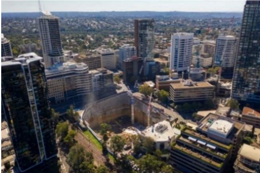
Figure 1. Aerial view of the excavation showing adjacent transport infrastructure
