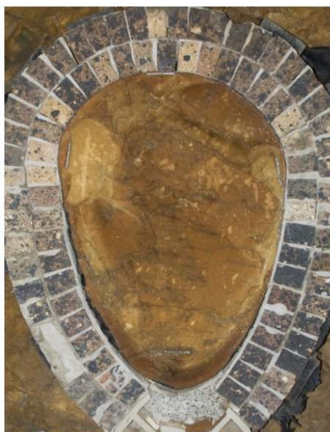
Figure 1. Typical brick oviform section (Source: Powerhouse museum)
