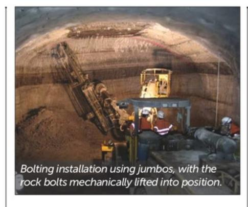
reinforcement (Pells, 2020) with strict controls that there is to be zero surface damage during construction. Modern day civil tunnels have shifted the focus to sustainability, cost savings and making the ground support itself. Rock bolts are now being designed to support the weight of tons of rock AND have a 100-year design life, double corrosion protection, fire resistance, be testable insitu and have the ability to withstand the impacts of seismic activity.
